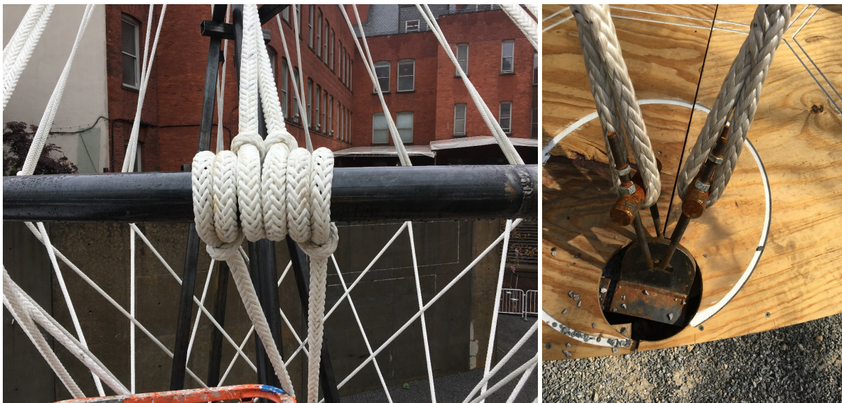
Figure 7: Rope connection at ring (left); rope connection at base (right)
